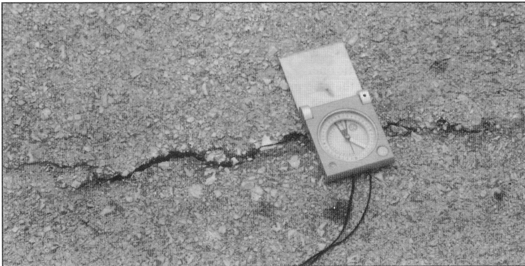
Fig. 7. Earthquake fracture on the road to Sarakina. Strike is N 100° E. Note the 2 mm right-lateral displacement of gravel, at the middle of the photograph.
